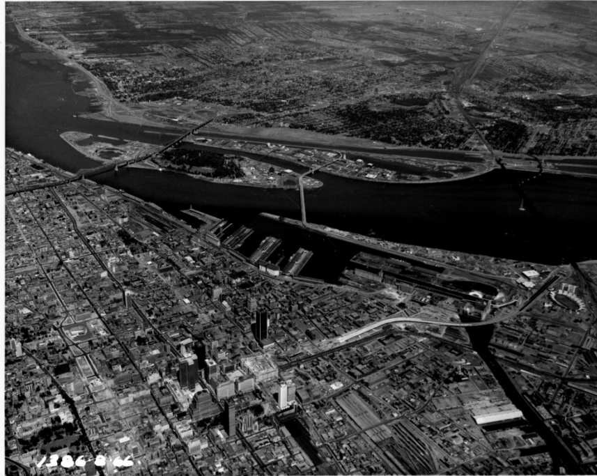
Figure 4. Expo 67 Site After Construction. 1966. Private Collection of the Author, Montréal
