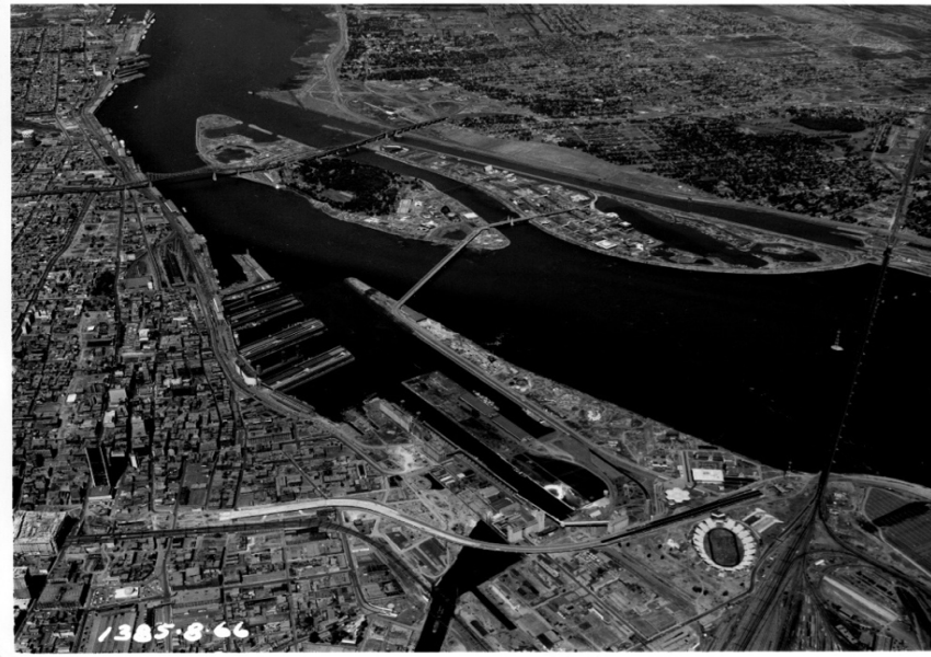
Figure 3. Expo 67 Site After Construction. 1966. Private Collection of the Author, Montréal
